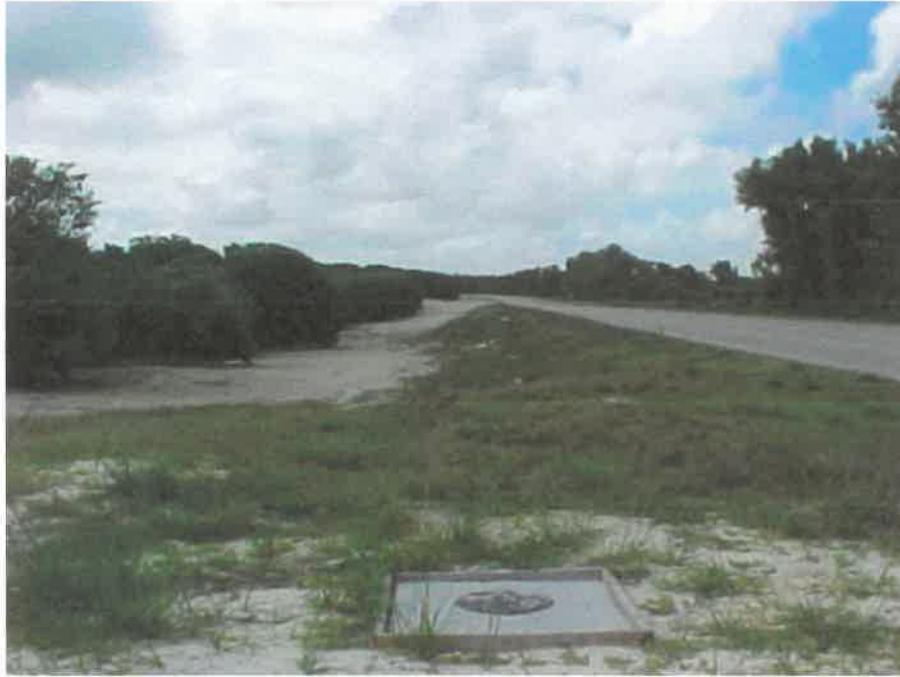
Figure 3: Typical appearance of a completed well at grade.
