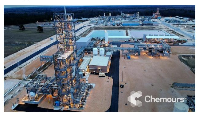
In addition to the thermal oxidizer, Chemours installed carbon adsorption units at other parts of the facility to control additional emission sources, on a compressed time schedule beginning prior to the Consent Order. Collectively, the thermal oxidizer, carbon adsorption units, and other measures have reduced HFPO-DA air emissions from the facility by over 99% as compared to a 2017 baseline.
