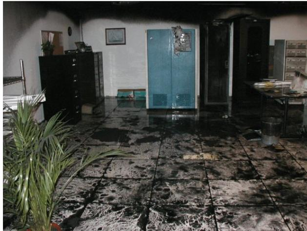
**Figure 2. Aftermath of pre-action sprinkler activation on an in-cabinet fire**
