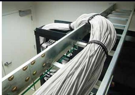
**Abandoned cable needs to be removed since it increases the fuel load of a building's concealed spaces.**
