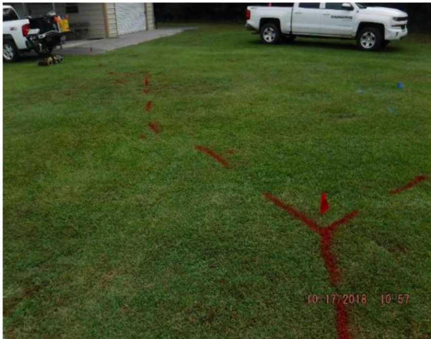
Red paint and flags marking underground electrical lines
