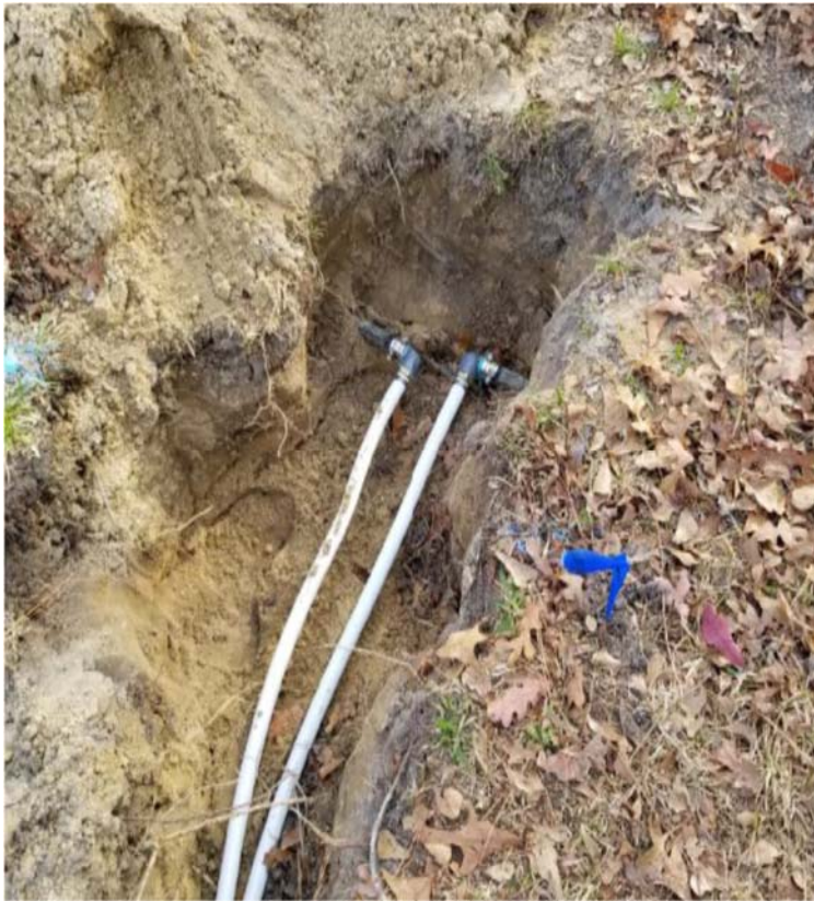
Example water line connection trench
